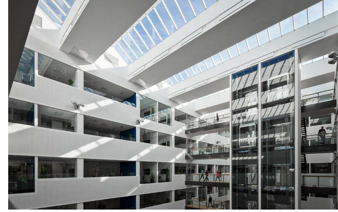
Shading in the atrium is provided by factory-fitted roller blinds that are automatically controlled according to for instance the position of the sun and the lux levels in the atrium.
