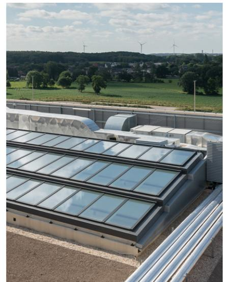
Even though our modules are rigorously tested and hold several fall-through certifications, VELUX Commercial do NOT recommend walking or stepping on the modules.
