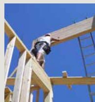
Structural beams being set to carry the SIP roof panels.
