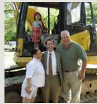
Matt Belcher, Active House project manager, and the Smith family just before demolition begins.
