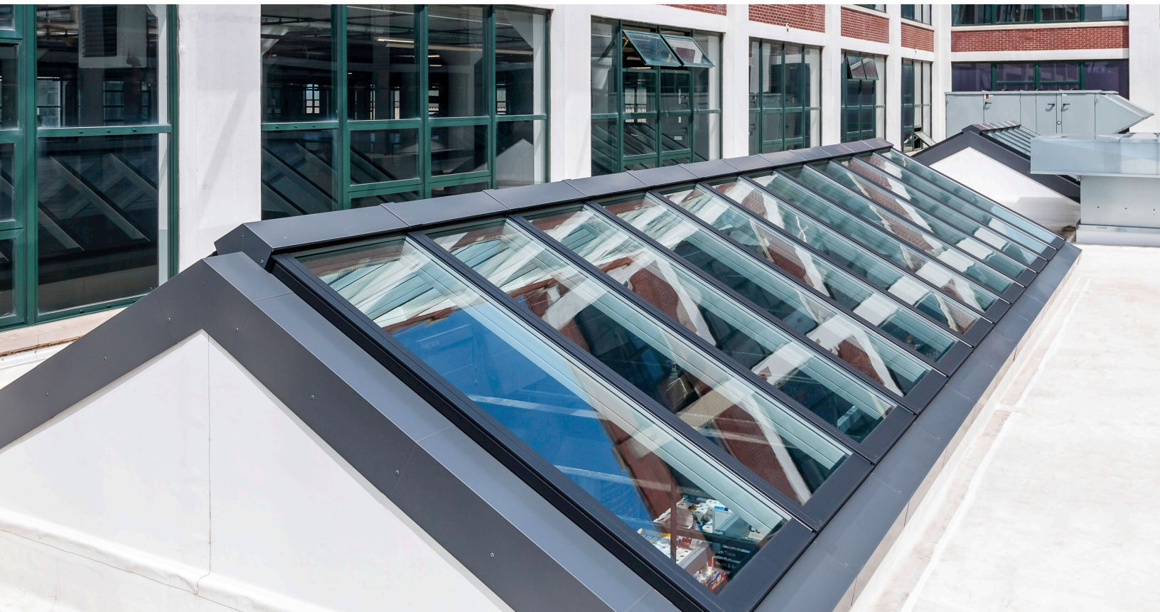
Skylights are essential to creating a pleasant shopping experience with natural light in this grocery store located on the ground floor.
