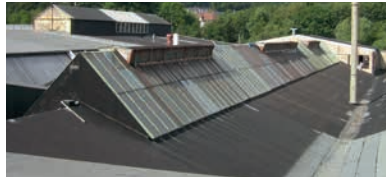
Wired glass saddle rooflight before refurbishment
