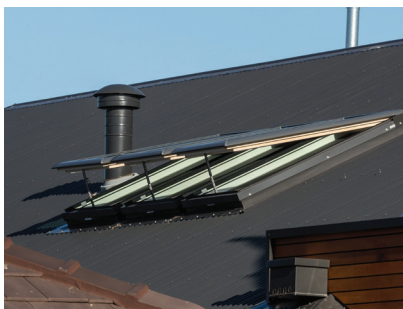
Pitched Roof Skylights
