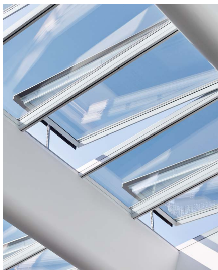
Glazing with electrochrome glass in clear state. Visible light transmission 57%
