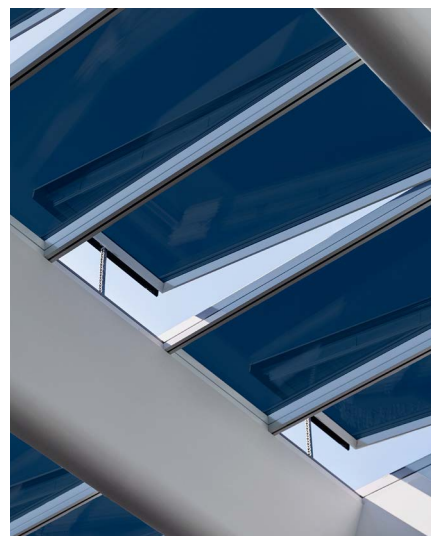
Glazing with electrochrome glass in fully tinted state. Visible light transmission 1%
