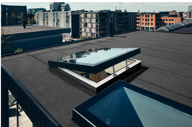
Connecting the electricity and checking the functionality
