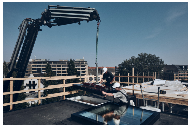
Placing the top unit
