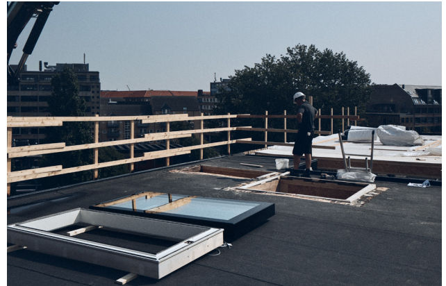
Preparing the hole for the upstand
