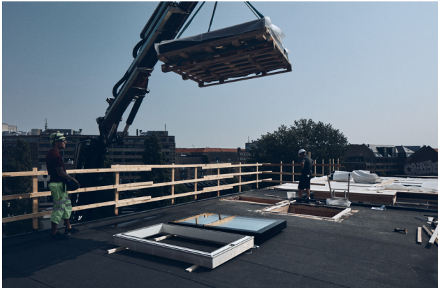
Craning products to the roof
