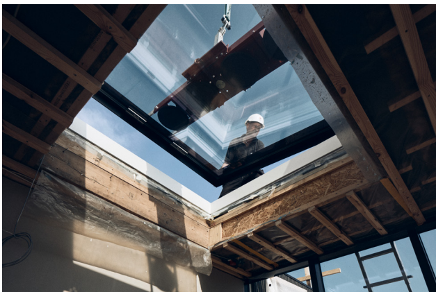
Placing the top unit
