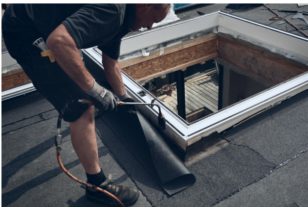
Securing the upstand and roofing material for watertightness without exposing the product to the flame.
