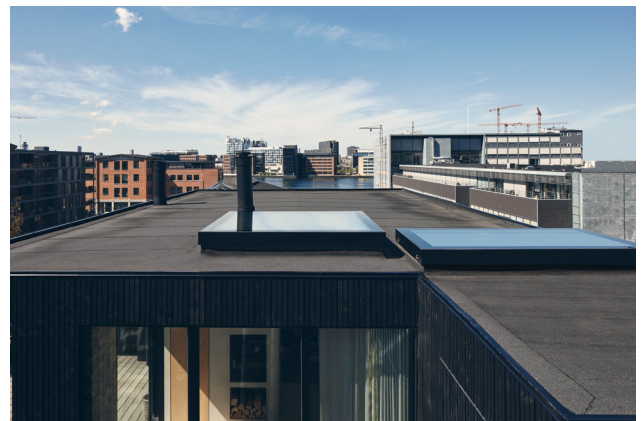
External work finalized
