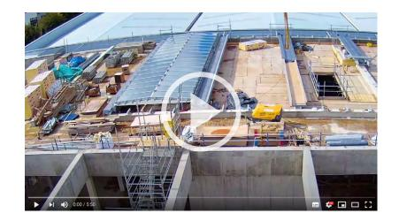
One of the Atria's was glazed in a morning, so the speed of installation can make the building watertight quickly and enable trades that are working inside to come onto site quicker.
