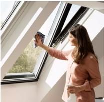
To clean the outer glass surface of the fixed window element from the inside, open the upper section fully to reach the outer glass surface of the lower section.
