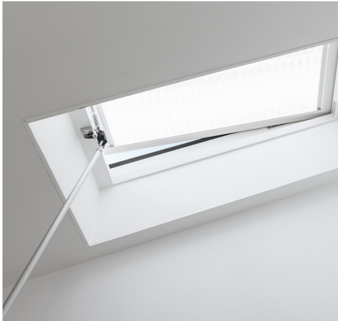
**Some artists initially found the high-level rooflights tricky to operate, but with the help of VELUX, hooks and rods were added, making the roof windows easy to open and close.**
