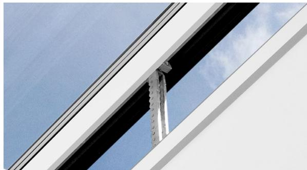
The hidden actuators open and close the venting units according to the remote controlled settings. Total integration ensures a discrete result.
