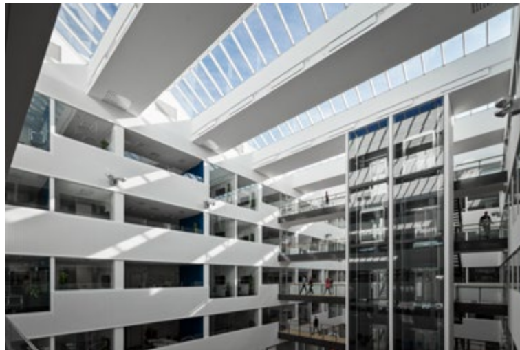
Siemens Head Office (DK) – LEED rating 'Gold'
